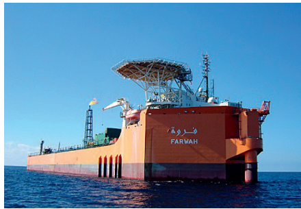
FPSO FARWAH, TOTAL
