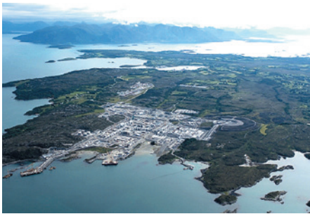
ORMEN LANGE, ONSHORE, SHELL
