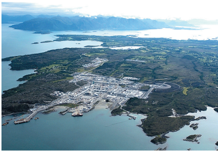
ORMEN LANGE, ONSHORE, SHELL
