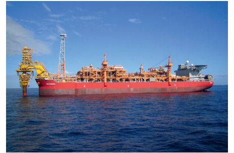
ENFIELD FPSO, WOODSIDE
